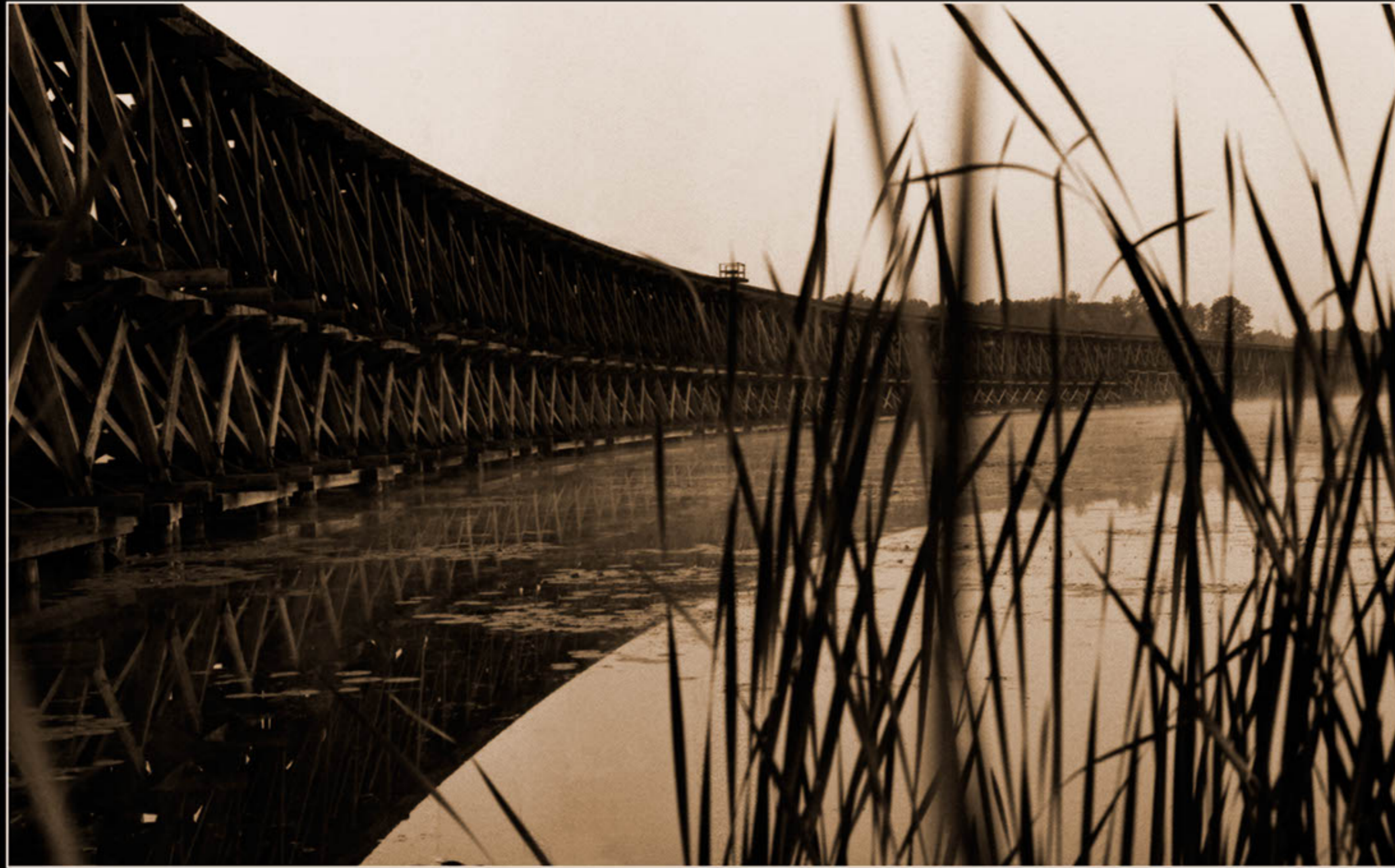
Hog Bay Trestle, Port McNicoll 1908-1978
